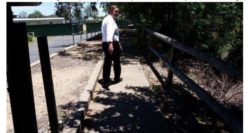
Shared path to Readford St (needs widening & connection to new bridge)
