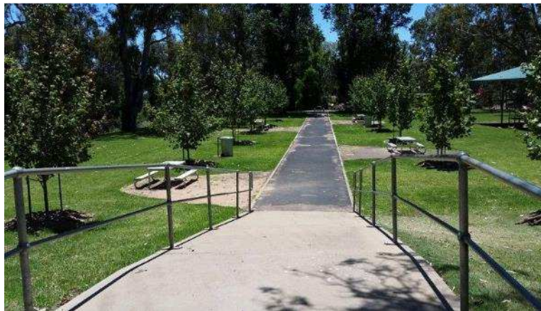
Repair pathway / accessible entries to seating areas
