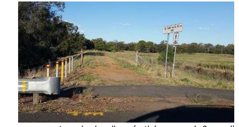
Levee bank walkway/path (spray, grade & gravel)
