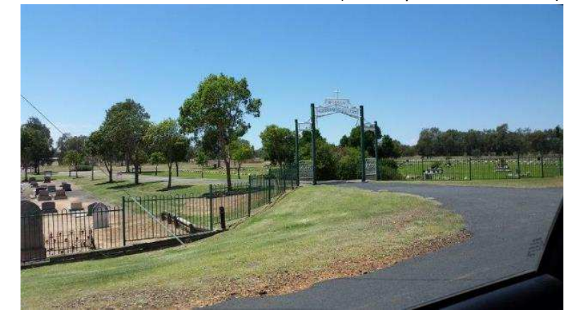
General Cemetery – Industrial Access Rd (Upgrade Chinese Section)
