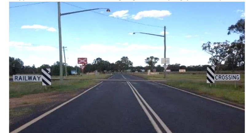
Warren Rail Line Crossing (traffic calming/future signalisation)
