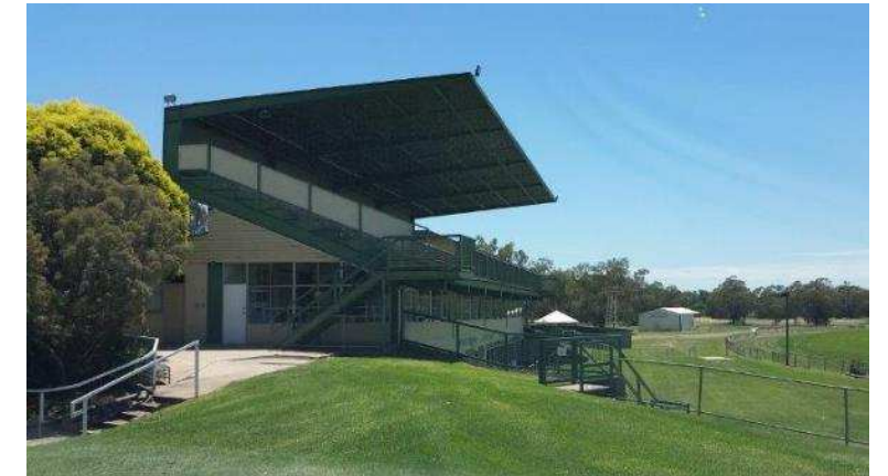
Racecourse stands (see list of improvements)
