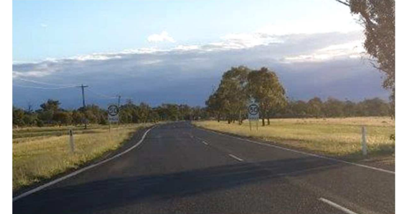
'50km/hr ahead' signs (limited visual cues for traffic calming)
