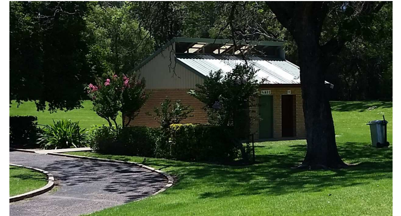
Toilet block (check accessibility / signage)
