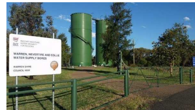
Warren Water Tanks – Ellengerah Rd (recent upgrades)
