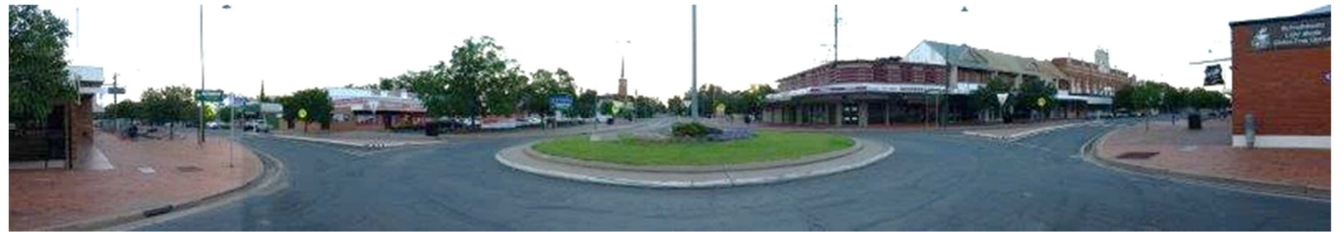
Oxley Hwy/Dubbo St Roundabout (needs to be focal point and provide navigation without clutter/safety issues -see Masterplan)
